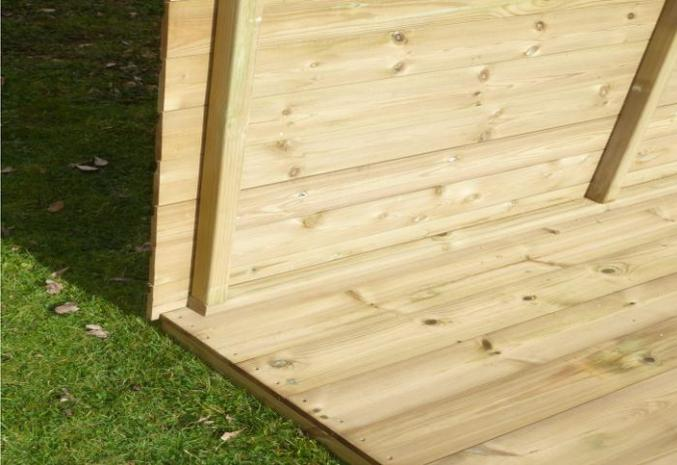
1. Place the floor section on the base you have prepared and fix the back panel to one side panel screwing through the vertical battens of the back panel into the battens on the side panel (3 screws). Repeat when fitting the other side panel (3 screws).
